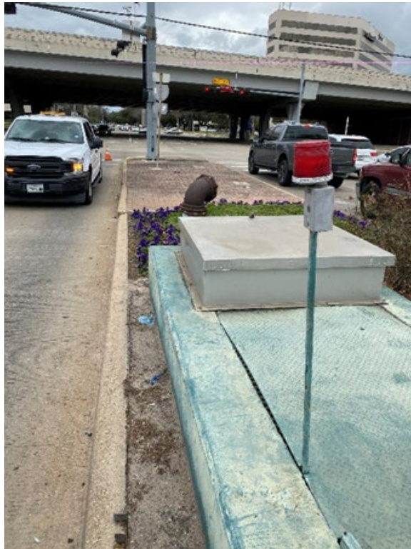
Figure 1-4. Bellaire Lift Station Street View
